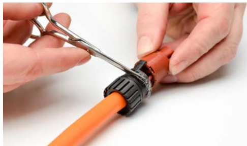
Step 14 - Trim shield as shown
