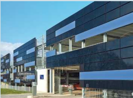
Building-integrated photovoltaics (BIPV)
