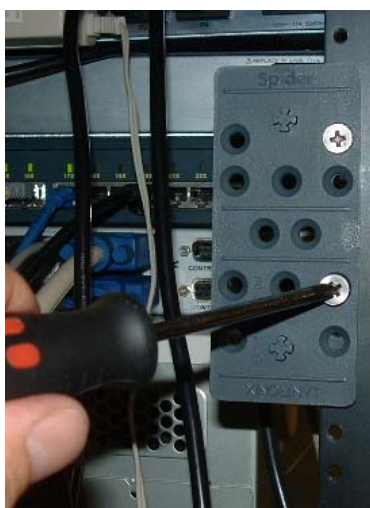
1. Mount the bracket with a Phillips-head screwdriver
