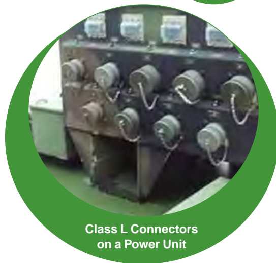
Class L Plug and Receptacle
