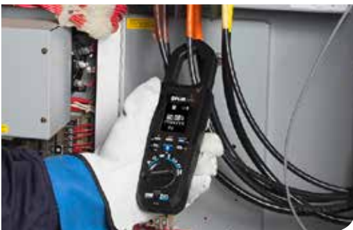
Verify amperage measurements
